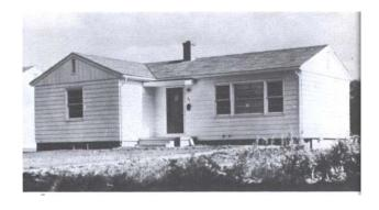
The porch is a later addition, as can be seen from the way it meets the siding on the front of the house and the house's foundation. However, it has form markings in the side of the concrete, indicating that it is an early addition.
