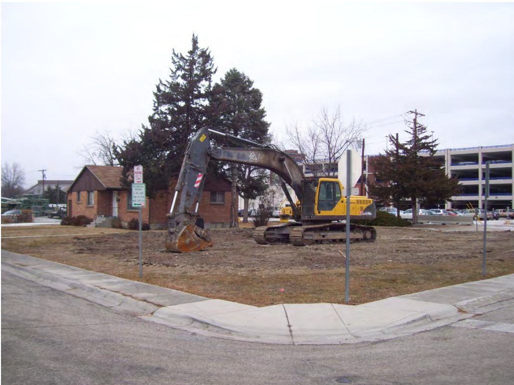
Photo 06: Belmont St. & Oakland Ave. Intersection – Looking North East
