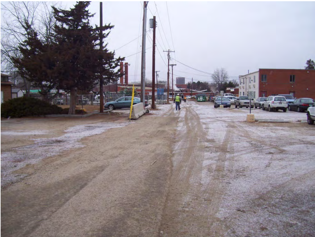
Photo 04: Belmont St. Mid-Block – Looking North
