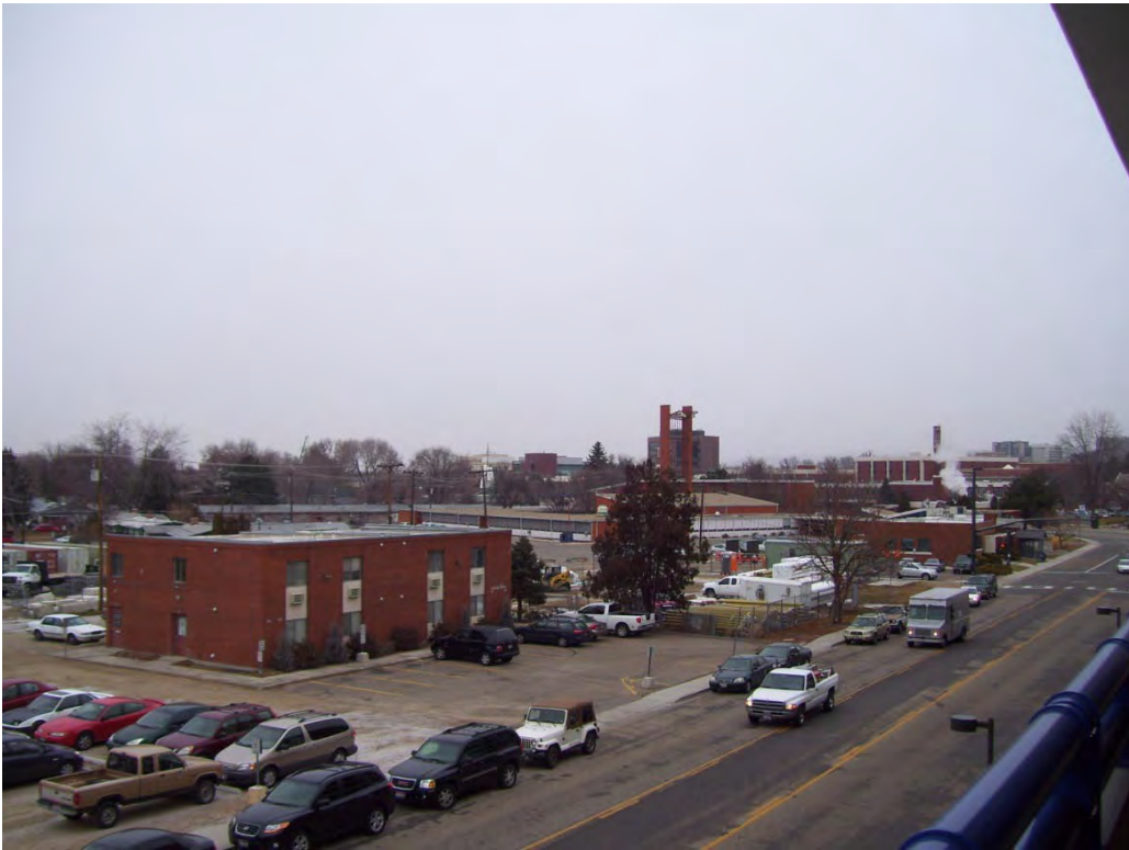
Photo 21: Lincoln Ave. Parking Garage Roof – Looking North West
