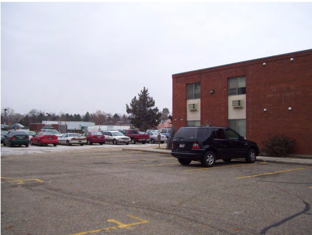
Photo 16: Lincoln Ave. Mid-Block – Looking South West
