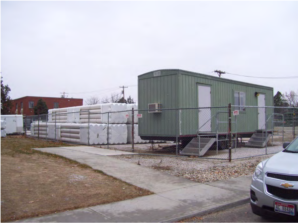
Photo 14: Lincoln Ave. & University Dr. Intersection – Looking South West
