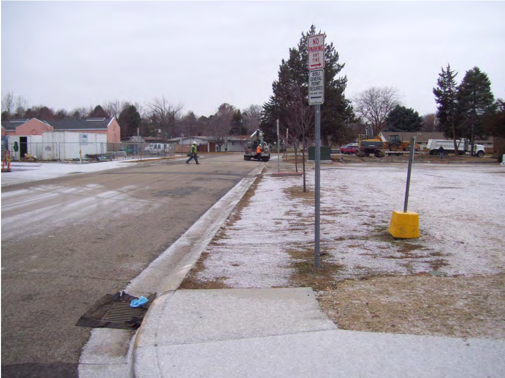
Photo 03: Lincoln Ave. & Belmont St. Intersection – Looking West
