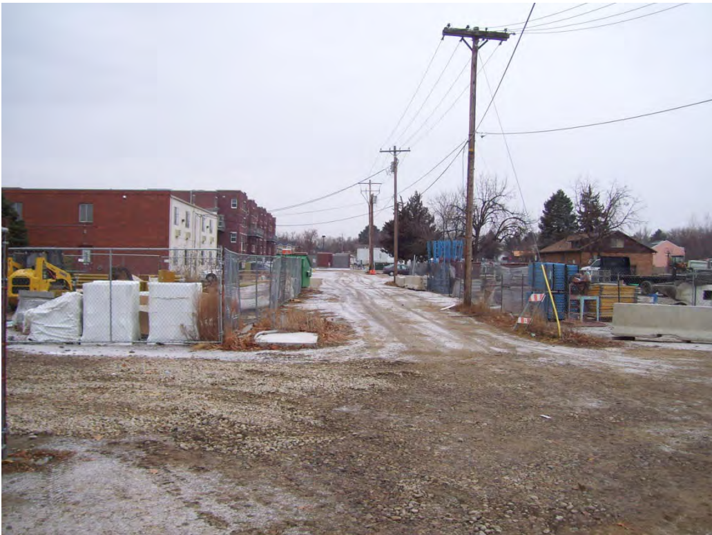
Photo 10: North Edge of Site – Looking South
