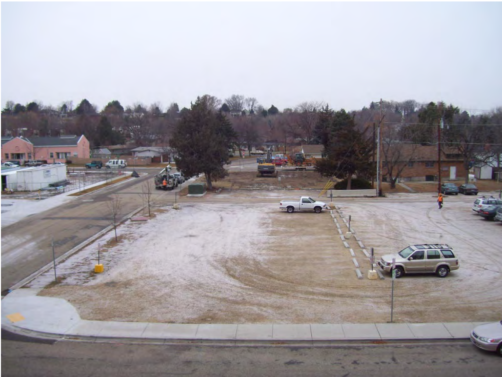
Photo 19: Lincoln Ave. Parking Garage Roof – Looking West
