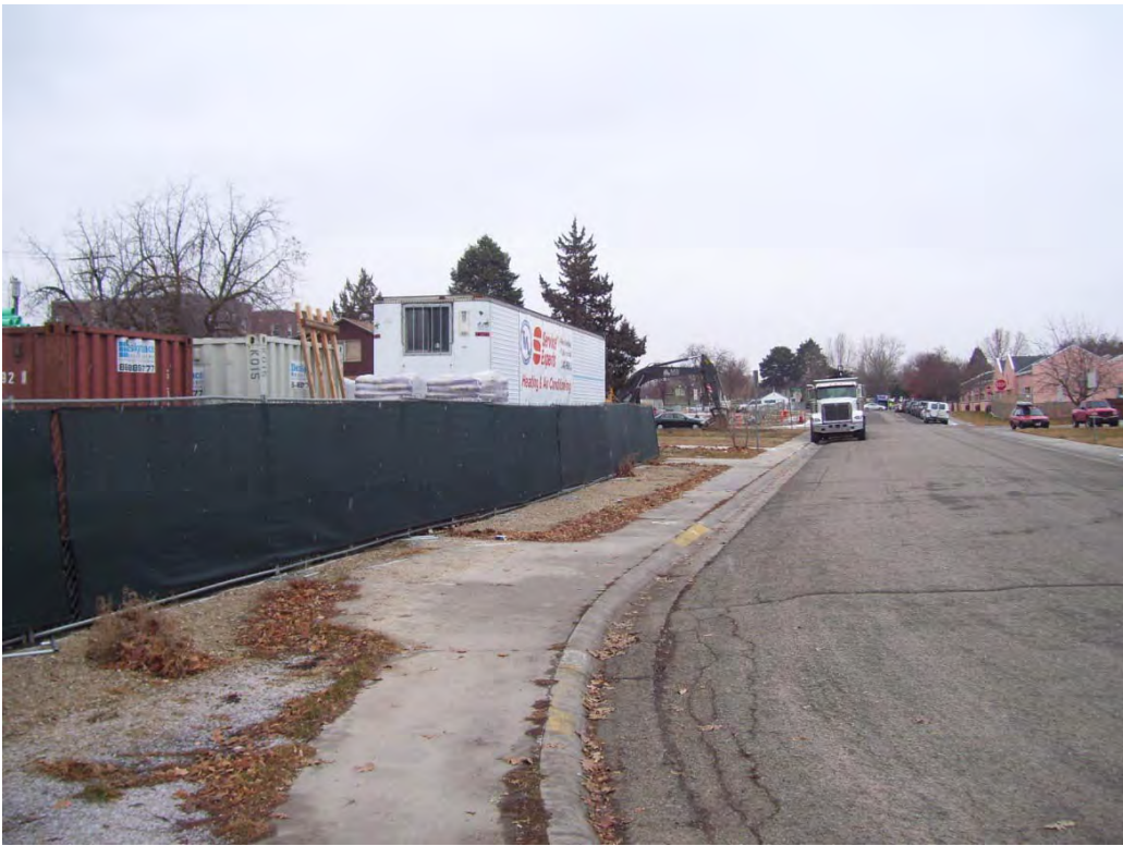
Photo 08: Oakland Ave. & Potter Dr. Intersection – Looking South
