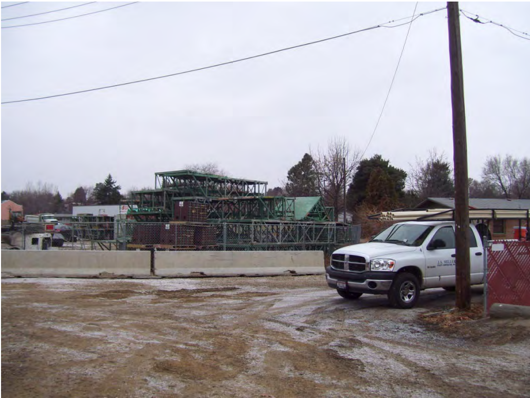
Photo 11: North Edge of Site – Looking South West
