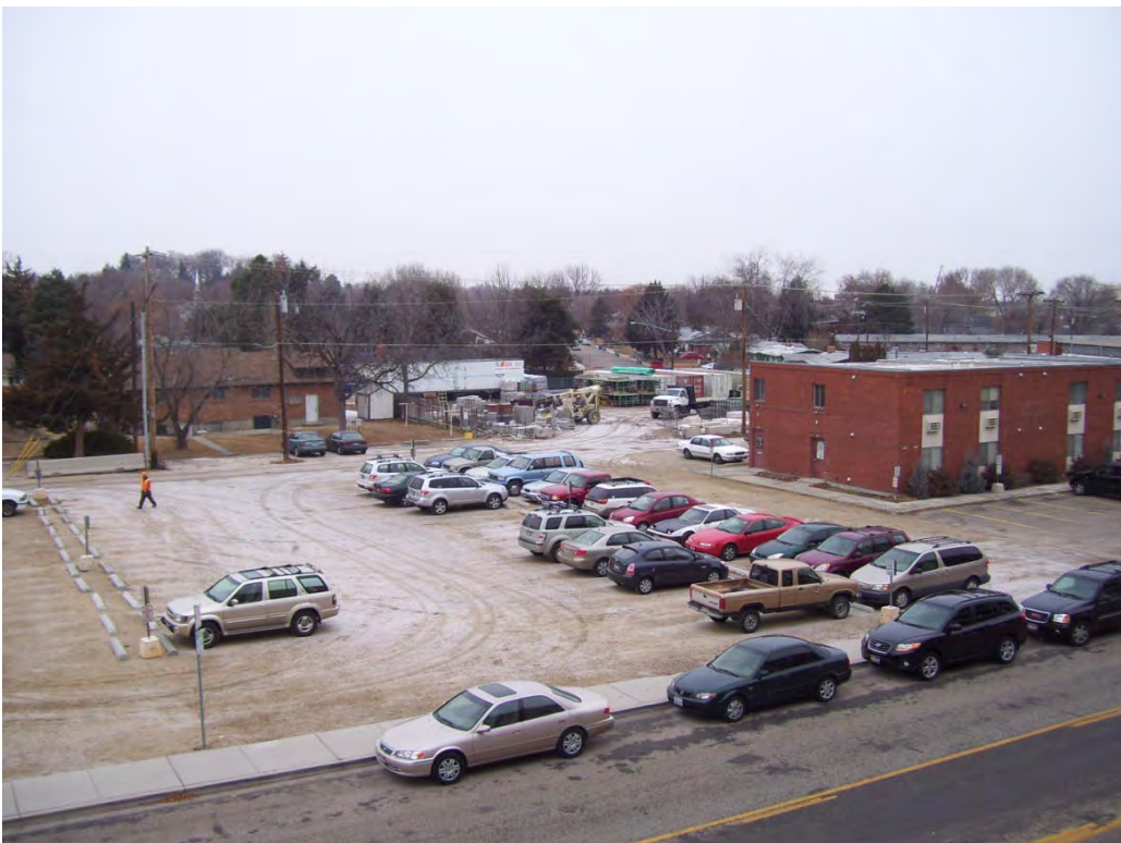
Photo 20: Lincoln Ave. Parking Garage Roof – Looking West
