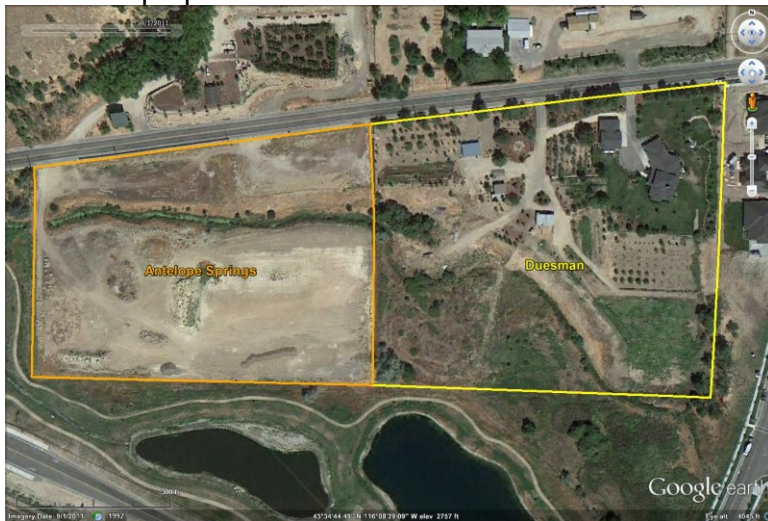
Figure 4. Antelope Springs and Duesmans (9/1/2011). As late as September 2011, the drain crossing both the Antelope Springs and Duesman property clearly remained open, while the remainder of the entire Antelope Springs had been extensively filled.
