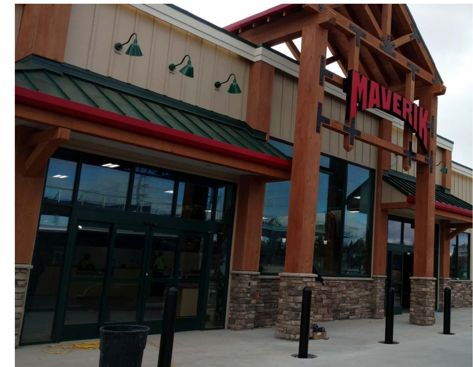
PHOTO OF EXISTING ADJACENT PROPERTY TO THE WEST LOOKING SOUTHWEST
