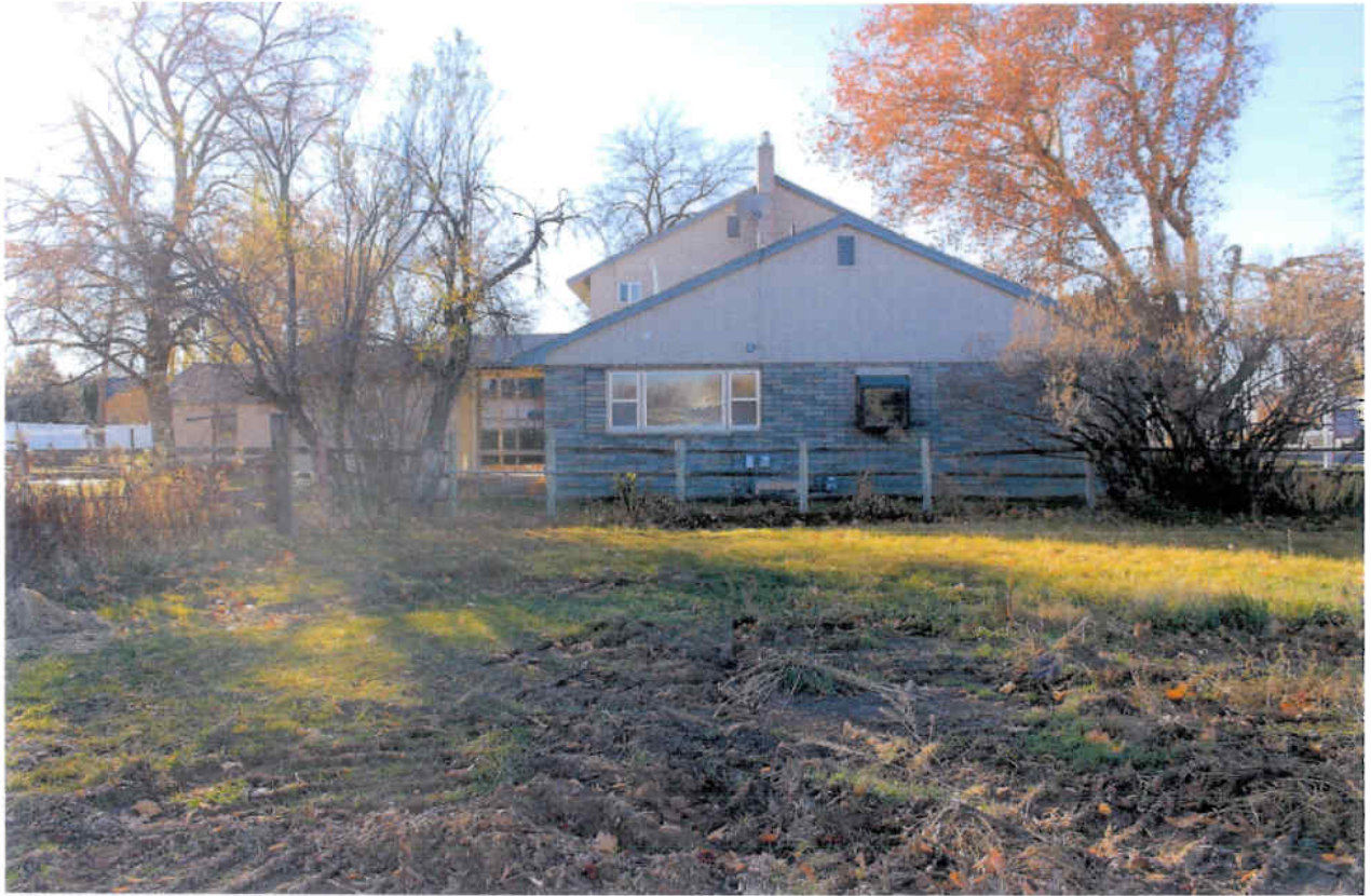
Figure 8: 2674 Mitchell looking South
