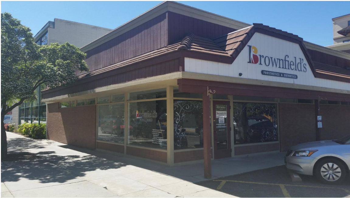
View looking South to Existing Building
