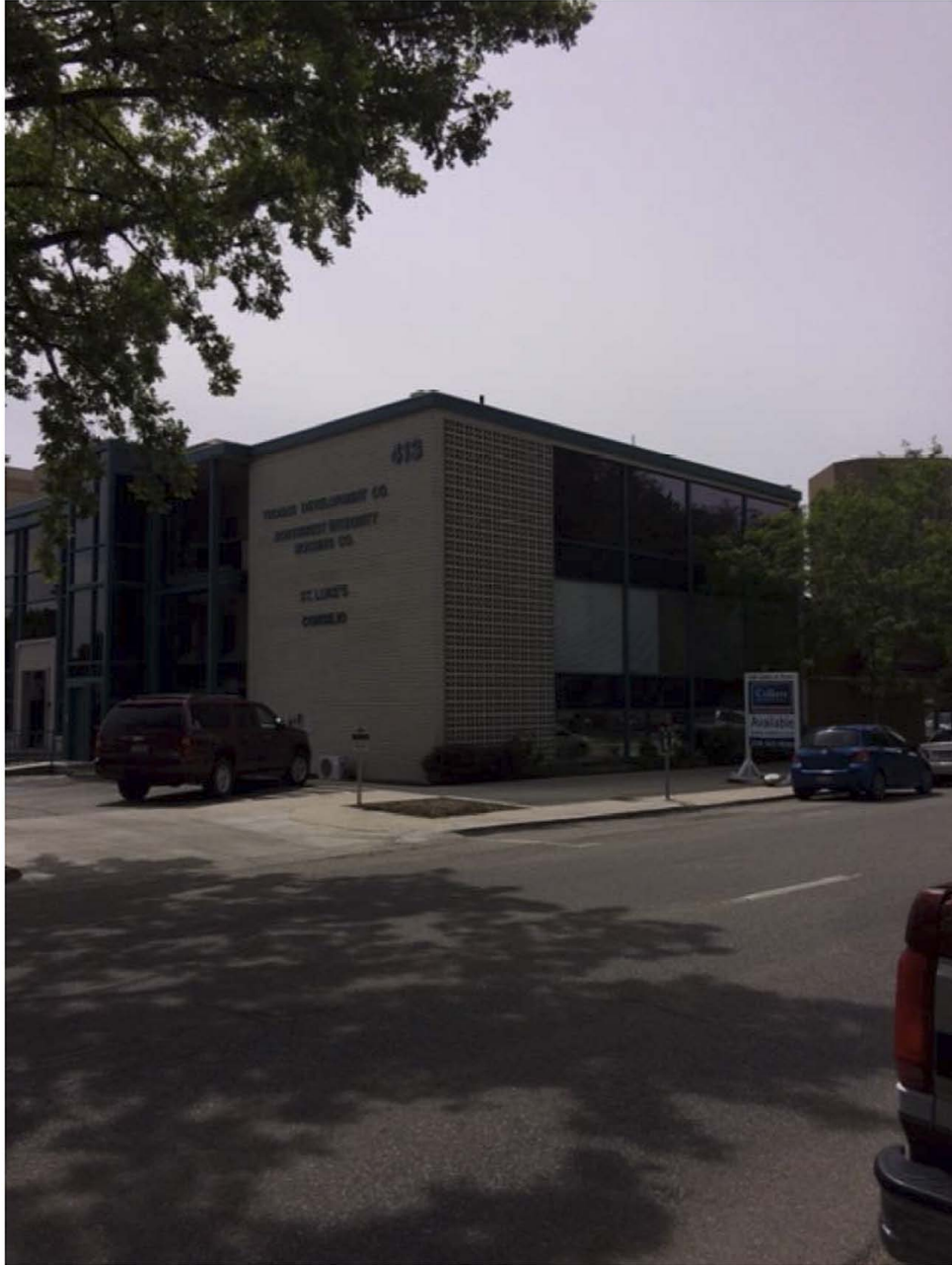
Adjacent building to east
