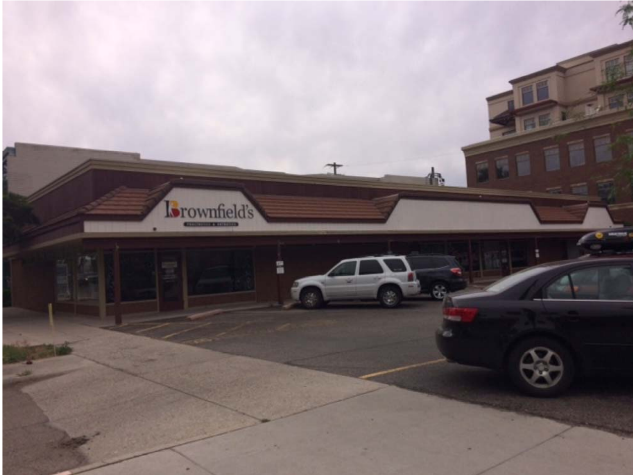
Front (east elevation) of building
