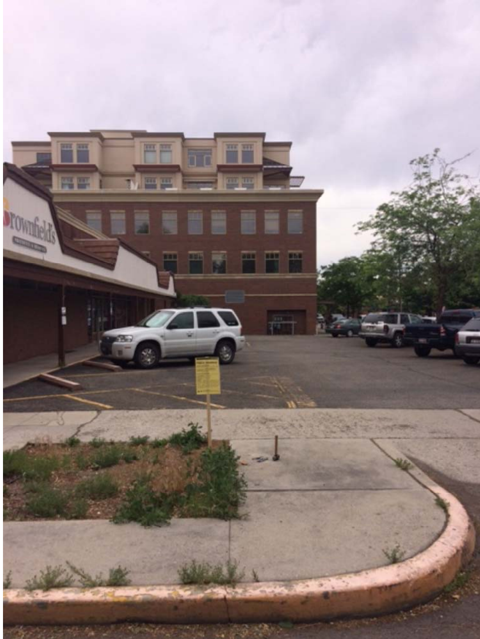
Parking lot from Idaho Street
