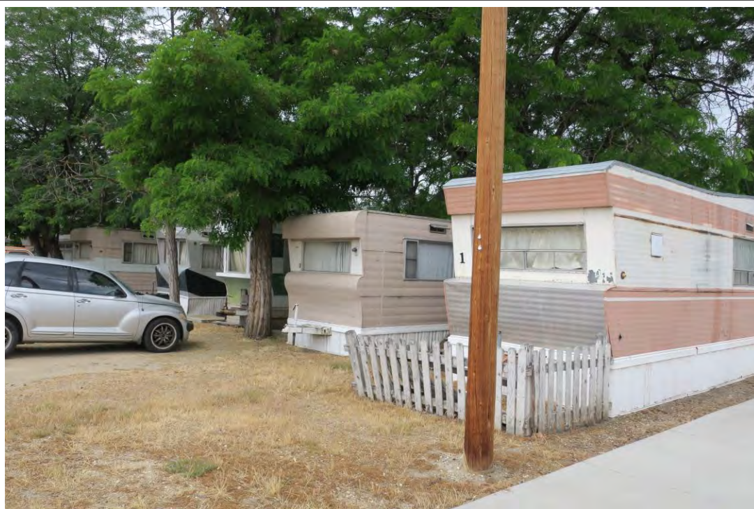
View SW of historic c1959 mobile homes, June 2017
