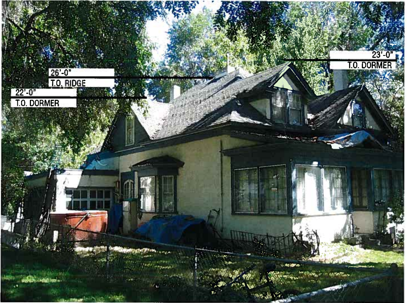
1614 N. 30th - 1 1/2 Story - Adjacent property south of project site
