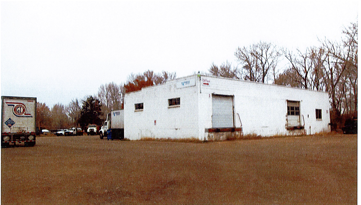
EXISTING STRUCTURE AT NORTHERLY BOUNDARY
