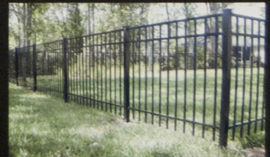
DECORATIVE METAL FENCE, GARAGE WALL OPENINGS
