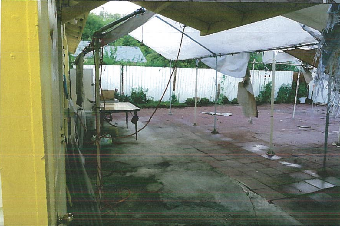
NEW BUILDING SITE
