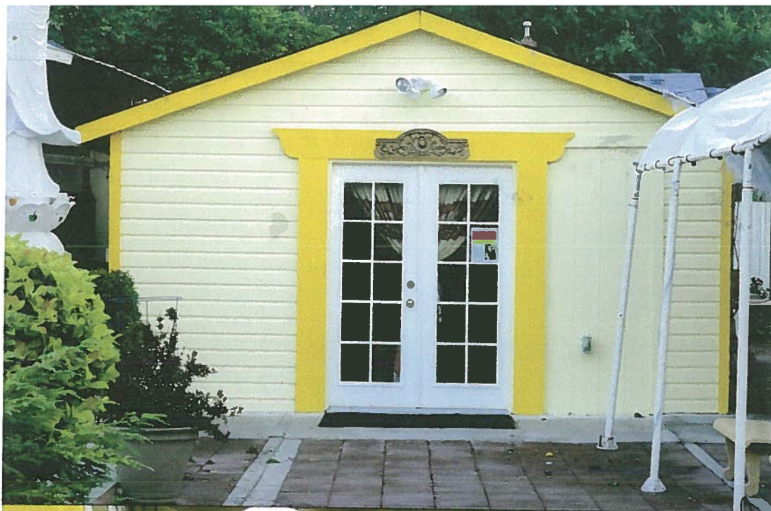
EXISTING BUILDING TO BE REMOVED
