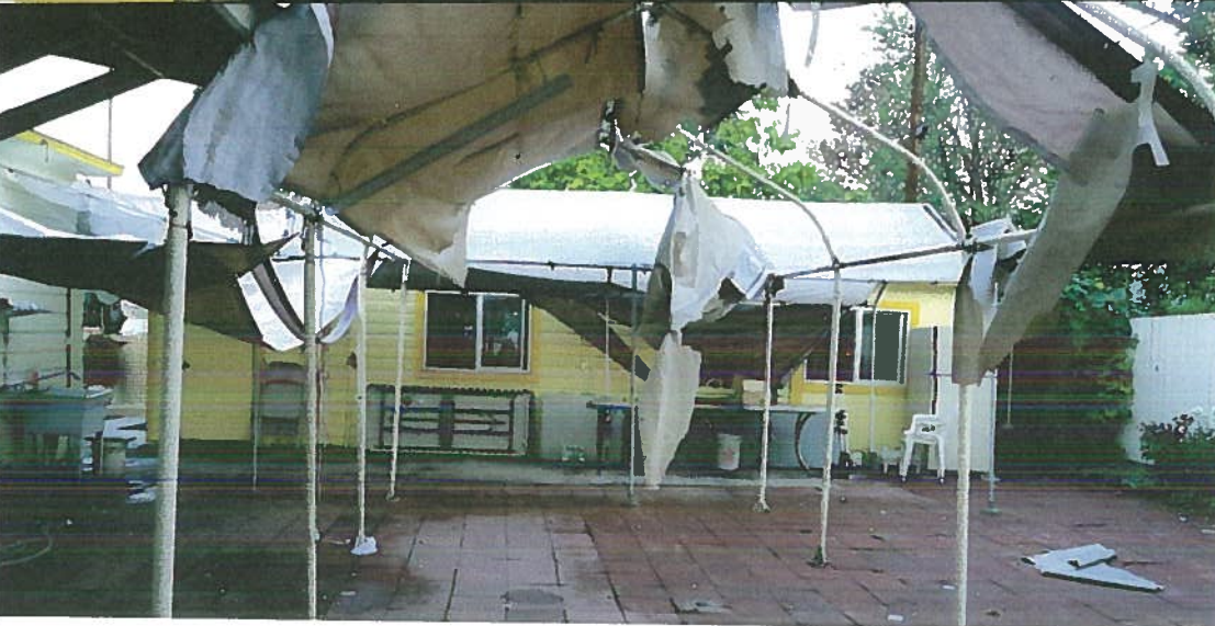
NEW BUILDING SITE
