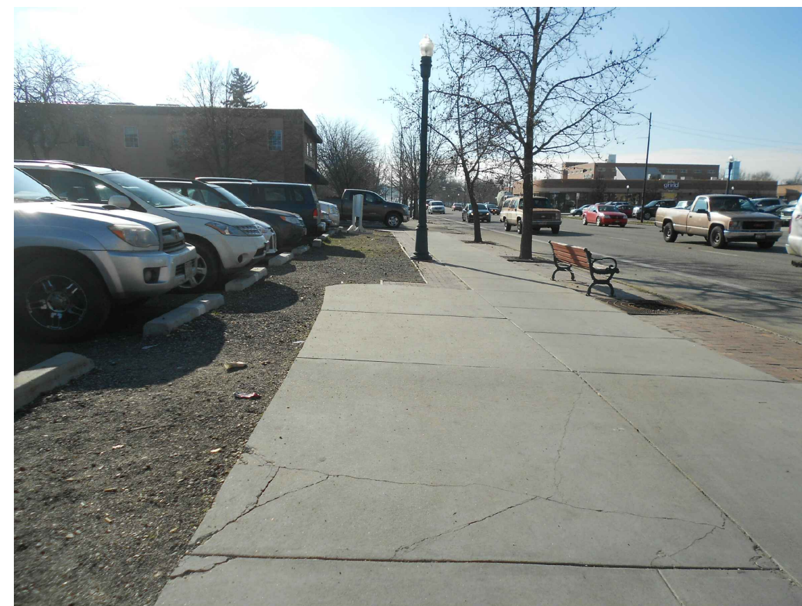
12 Looking south down Capitol Blvd.
