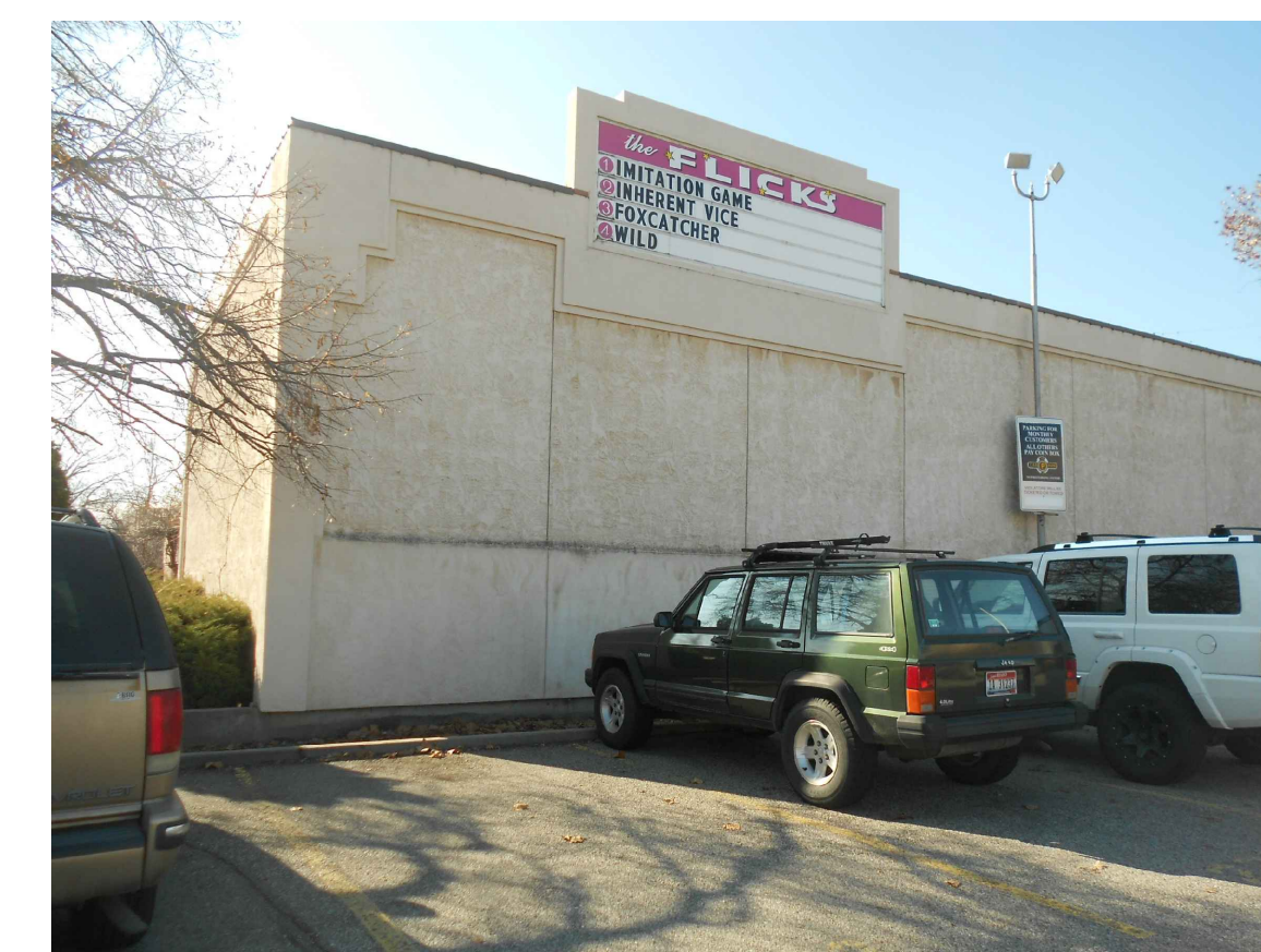
8 Existing Flucks theater to the south of proposed project site
