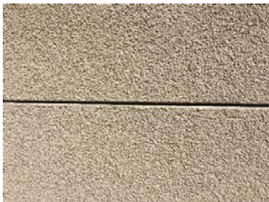
Upper stucco texture with reveal
