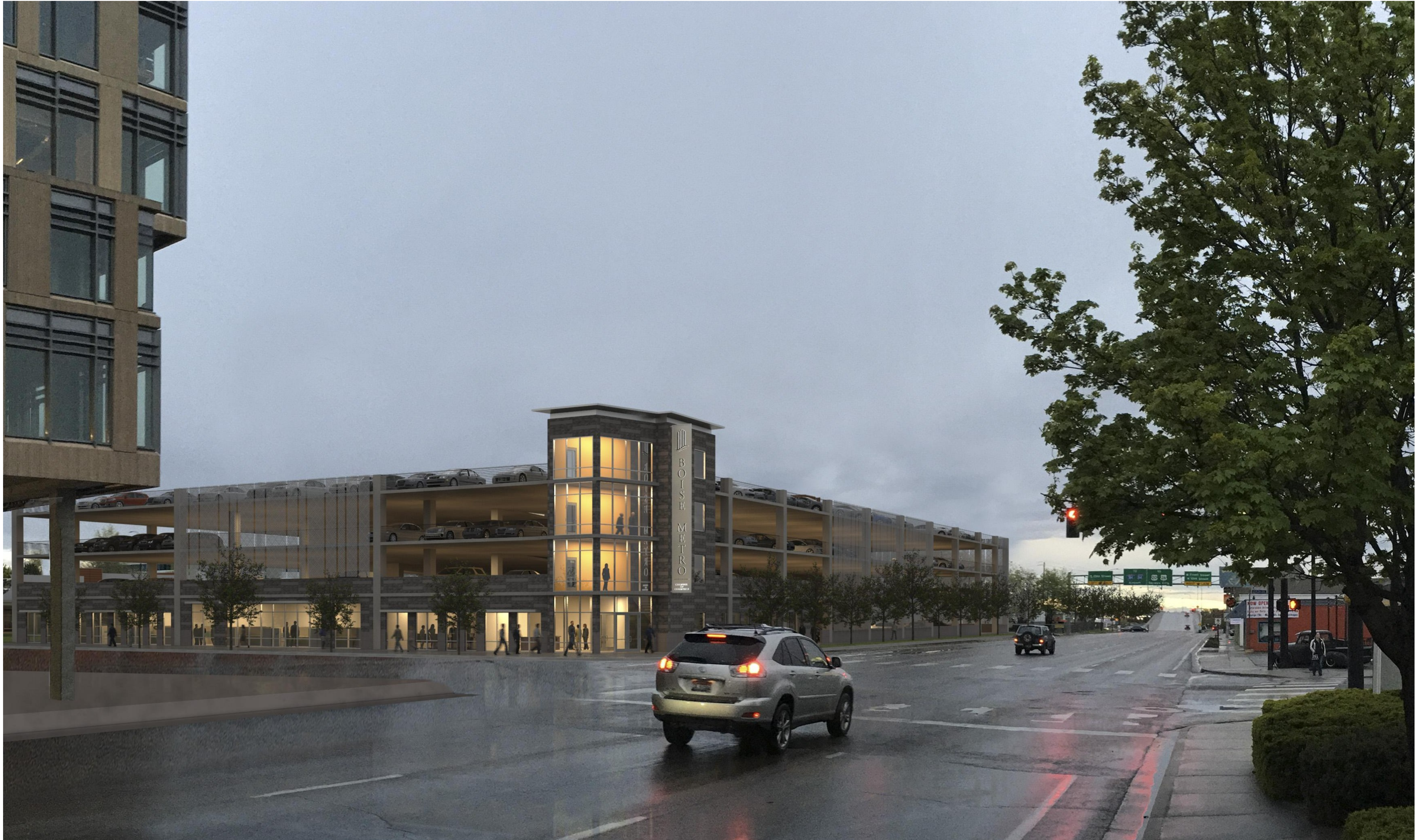
PARKING VIEW FROM FRONT & 11TH STREET
